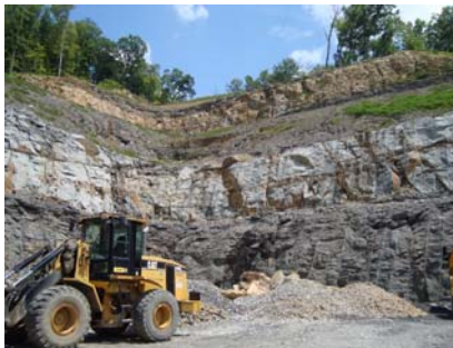
Portion of cut at the end of Phase I/beginning of Phase II
